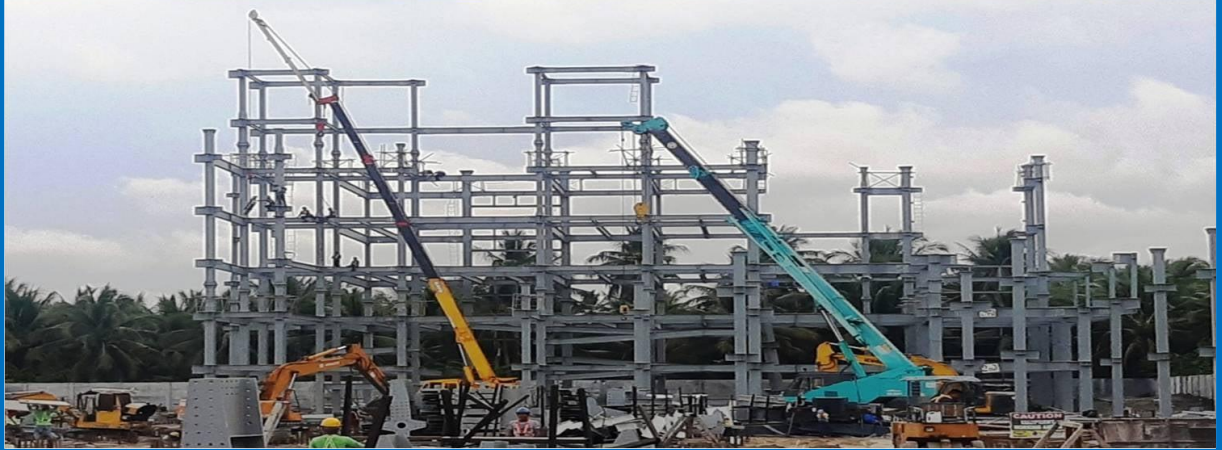
Project: ACE Hospital General Santos, Philippines
